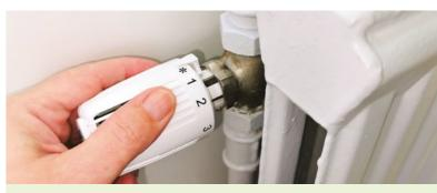
Each symbol 0 = Off  $3 = 20^{\circ}C$  on a TRV is a  $* = 7^{\circ}C$   $4 = 25^{\circ}C$  room temperature  $1 = 10^{\circ}C$   $5 = 30^{\circ}C$  setting:  $2 = 15^{\circ}C$
